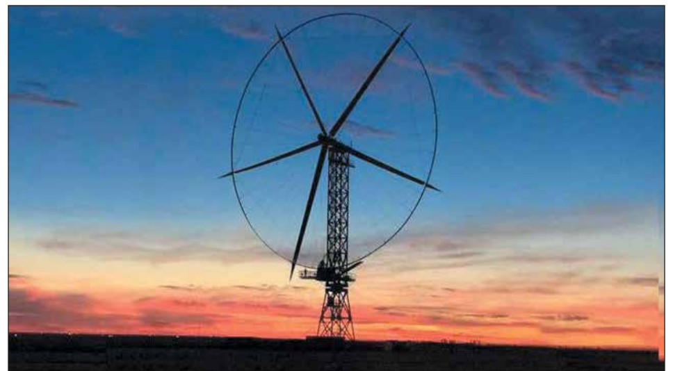
The 220-foot 800kW land-based prototype installed in Hooker, Okla., has evolved into the gen-2 BarberWind Turbines 800kW. Jerry Barber in this photo is standing on the generator platform. (Photo/Provided)
